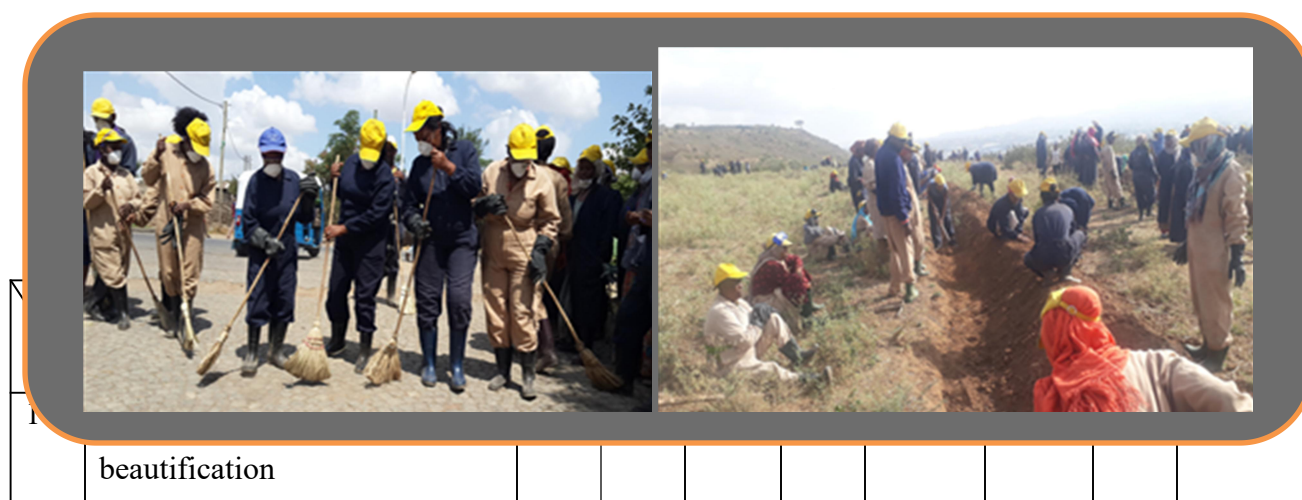
Figure 18:- Public works performed by UPSNP in Adama City
